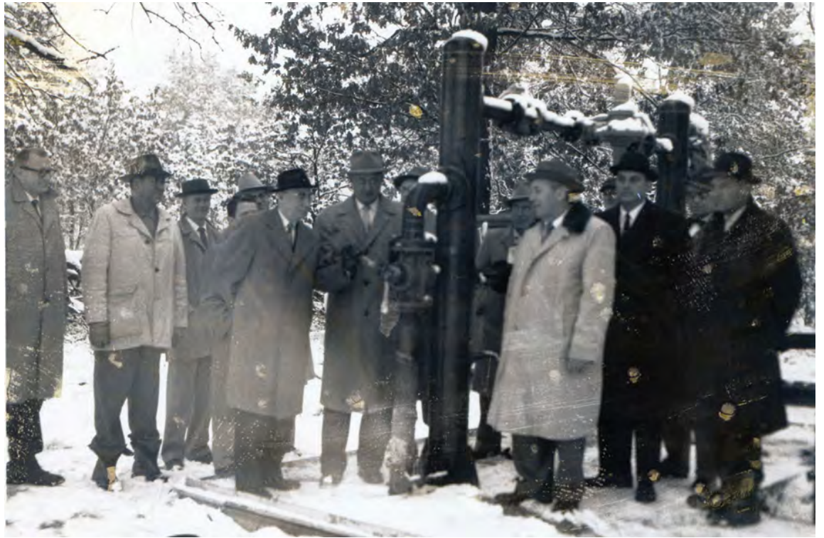
Turning on natural gas for Circle Pines in December 1959.
